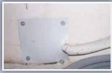
Power supply hole sealed with metal flashing.
